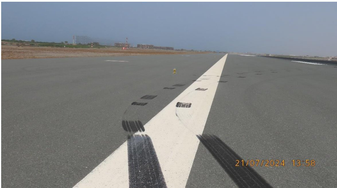
Figure 1: showing evidence of left main wheel tire marks outside the left edge of the RWY 08L.
