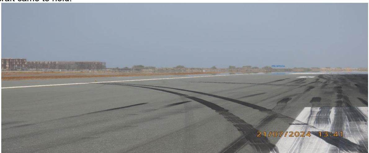
Figure 6: showing evidence of tire marks turning to the left of RWY 08L.
