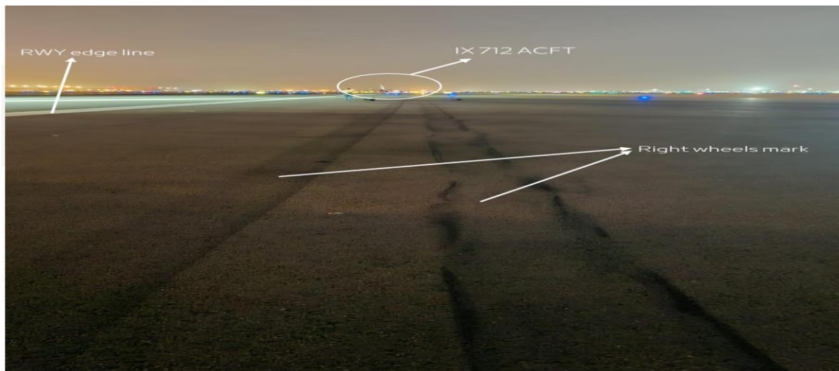
Figure 4: shows the tier marks on the right side of RWY26L (Source OA)
